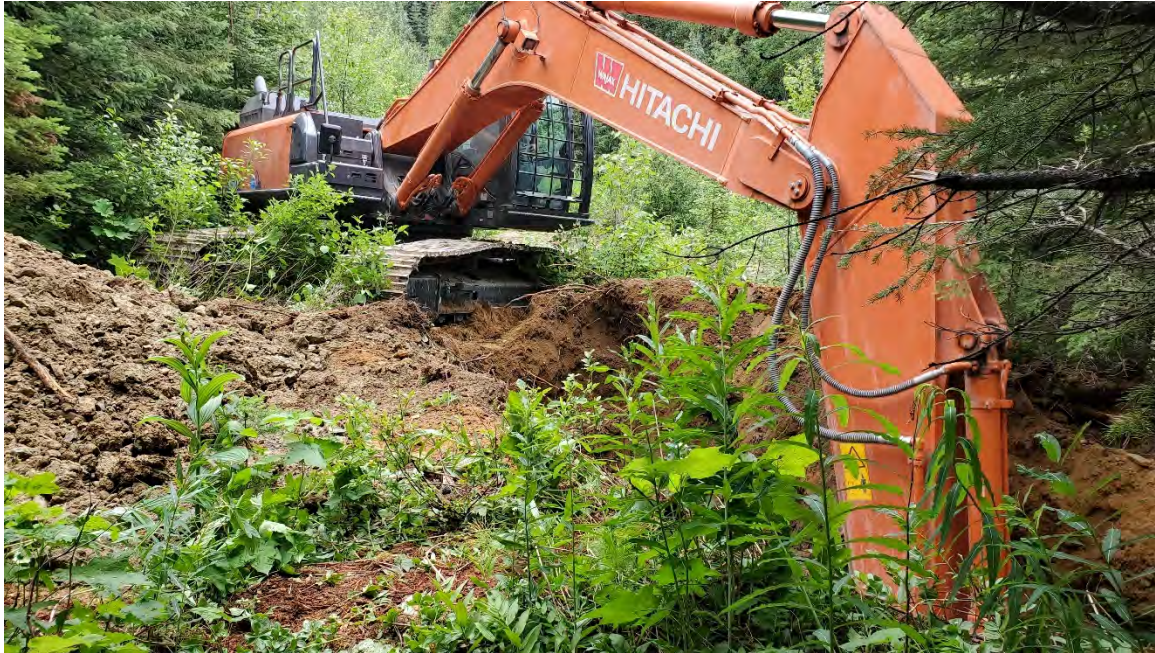
Image 2: Excavated test pit sampling underway
